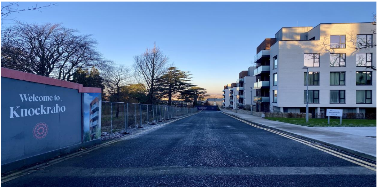
Figure 5: View from the site to the north looking along the edge of completed Phase 1 works.
